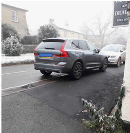
Photo C Looking westwards from junction with Duncock Lane with cars part parked on footpath and showing camber of footpath (11/12/22). Problem persists as shown at photos A and D.
