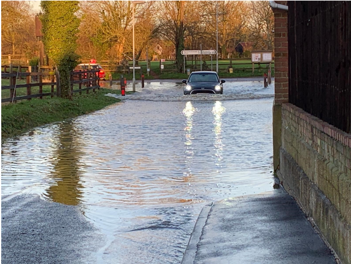
Local flooding outside The Poacher due to excessive run-off from Smith Street.
